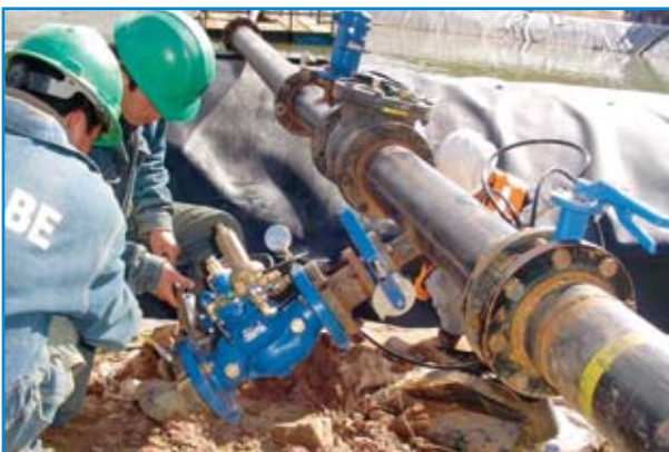
Corrosion-resistance safety valve, air and butterfly valves
