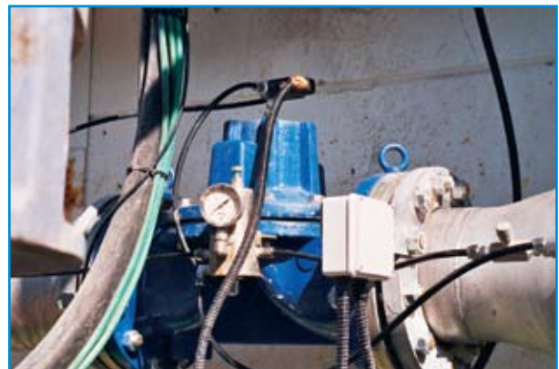
High pressure, electrically-controlled, corrosion resistant valve
