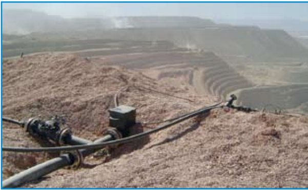
Pressure Sustaining valve, pipes flushing
